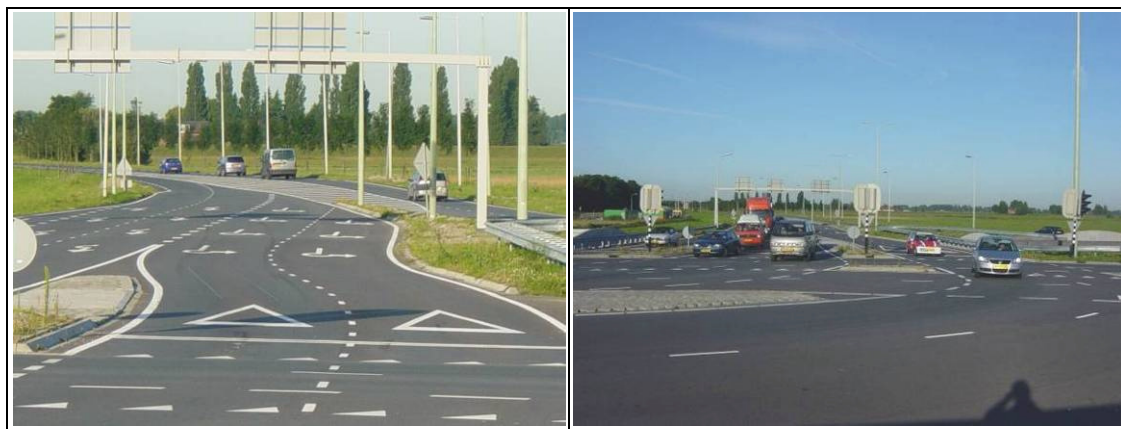
Figure 84: Example of signalized turbo roundabout (Doenkadeplein, the Netherlands)
