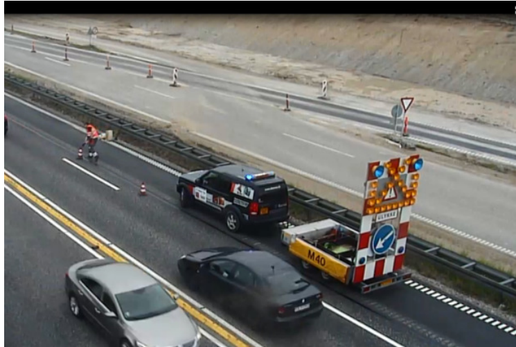
Lane closure on 4+0
