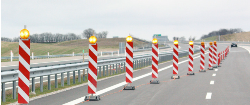
Lane closure taper/running light
