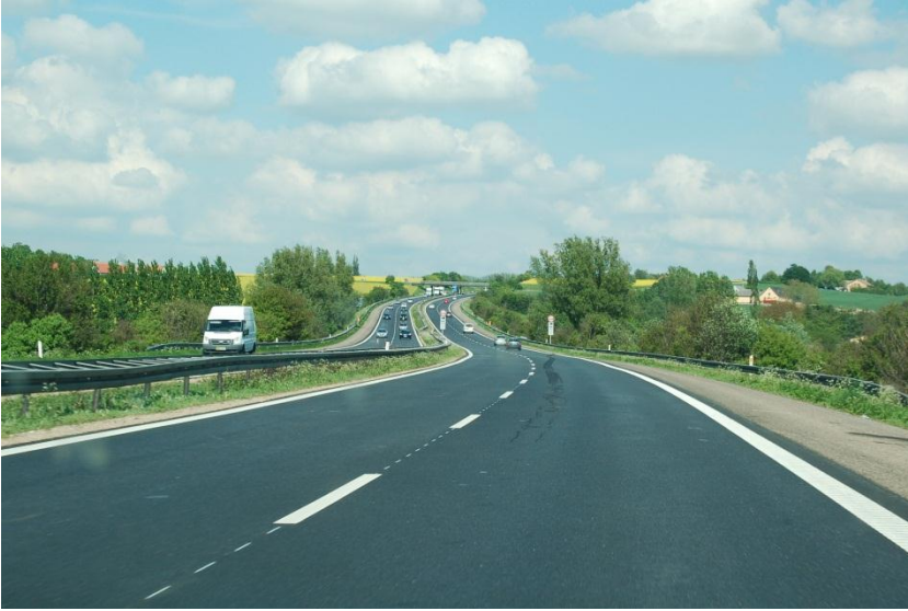
Figure 2: If the road is a national highway we expect the road standard to be relatively high.
