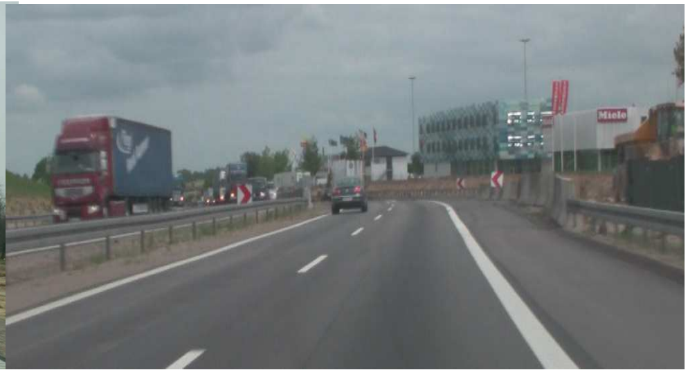
Interim motorway – high standard
