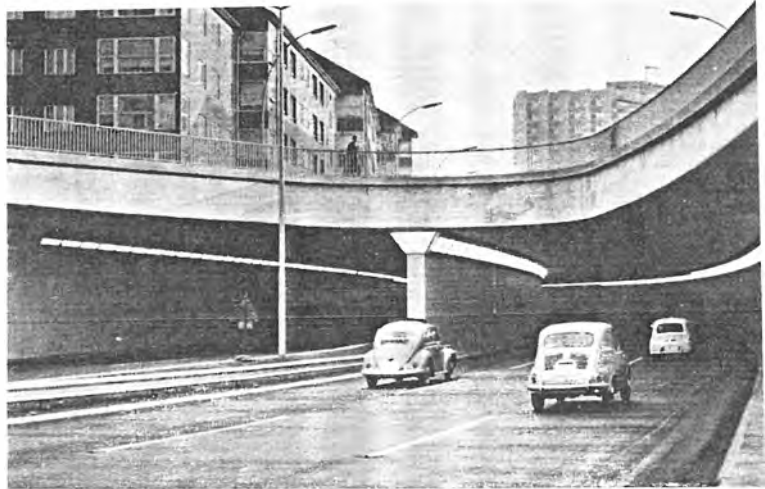
Plate 1. Optical guidance at a tunnel entrance.
