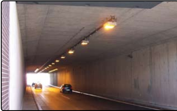
Figure 10: Combination of Lichtschleuse and supplemental daytime lighting in a tunnel in ‘Wolmirstedt’ (Germany)
