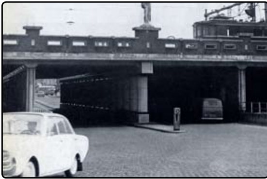
Figure 7a: One and the same tunnel can be regarded from one side as 'long'... (Source: Schreuder D.A. 'Short Tunnels'. International Lighting Review , Vol 16, No 3 (1965) p95.)
