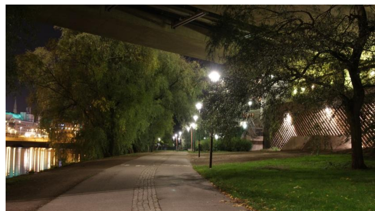
(Fig. 1.7) Photograph showing the lights washing the walls under the bridge
