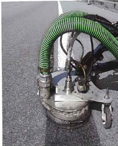
Waterblasting does not use harmful chemicals or damage the road surface in any way
