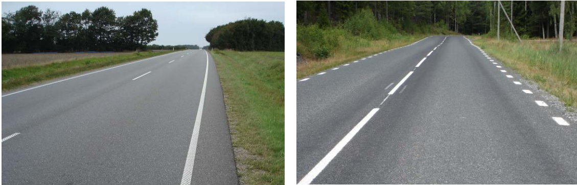
Figure 3 Typical test sections in Denmark and Sweden with continuous (left) and broken (right) edge lines.
