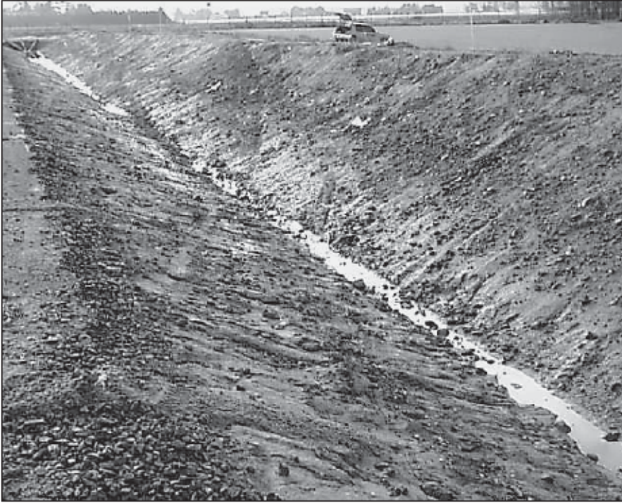
Figure 28 Tested V-ditch at Pori test site (FinnRA 2003).
