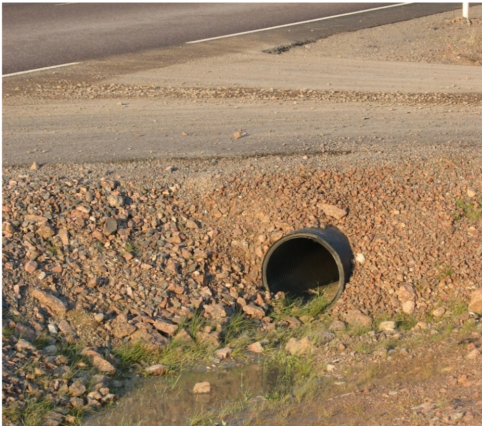
Figure 6 Parallel drainage culvert at recently built minor road junction (photo: Marko Kelkka)
