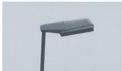
Figure 37: Some luminaires with weak cut-off in the classes G*1, G*2 and G*3.
