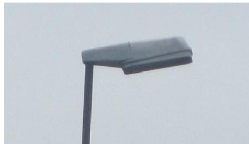
Figure C.19: Some luminaires with weak cut-off in the classes G*1, G*2 and G*3.
