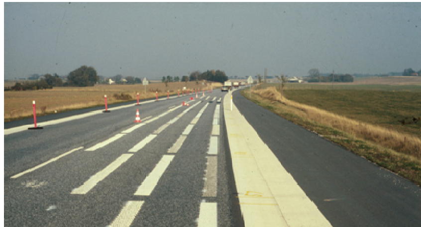
Figure A.10: Road markings on a test road seen with the sun
