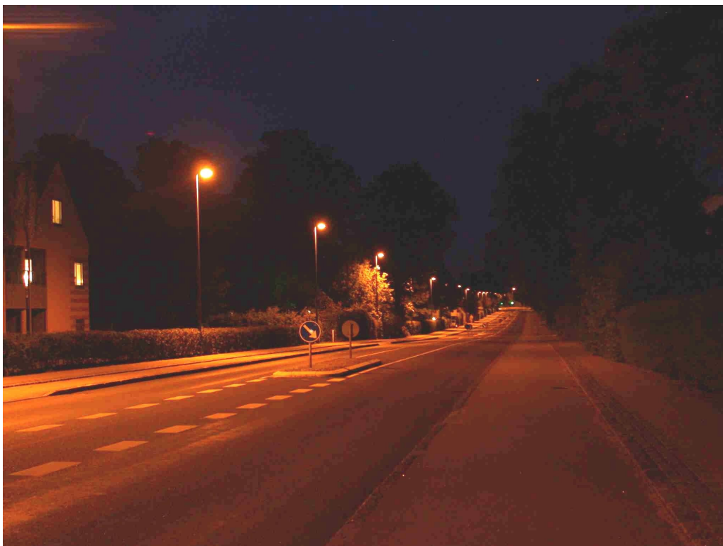
Figure 8: A typical road lighting installation on a small traffic road.
