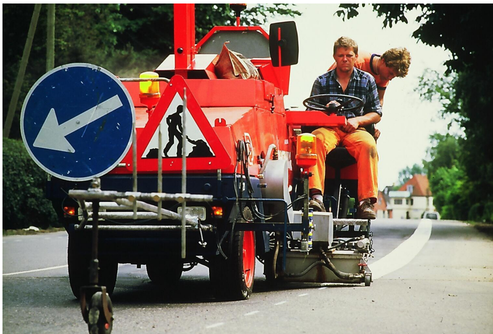
Figure 1: Machine application of an edge line.
