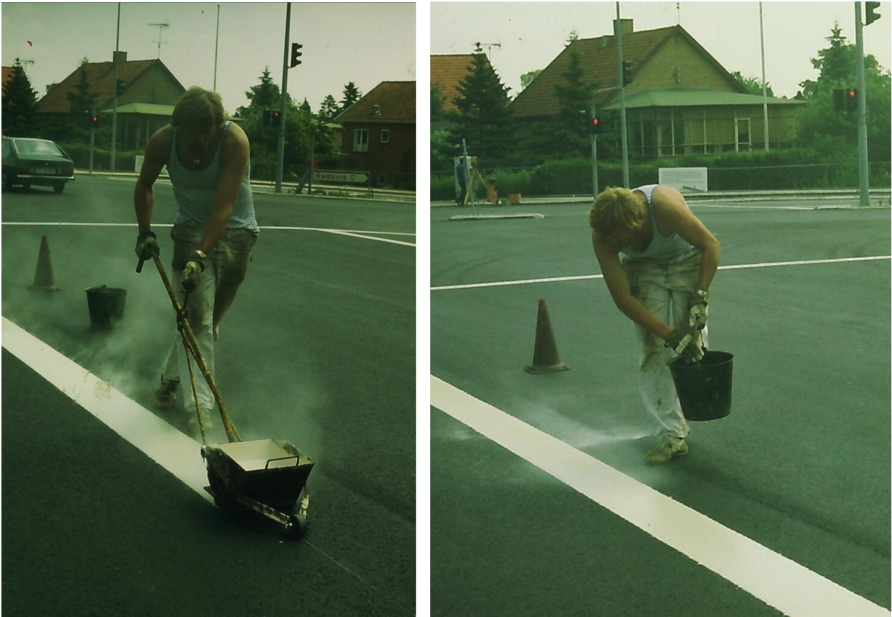
Figure 2: Application of thermoplastic by hand followed by spreading of glass beads.
