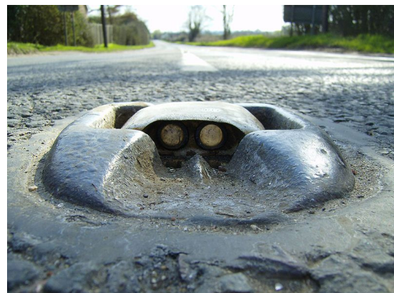
Figure A.5: Two cats eyes mounted in a road stud.
