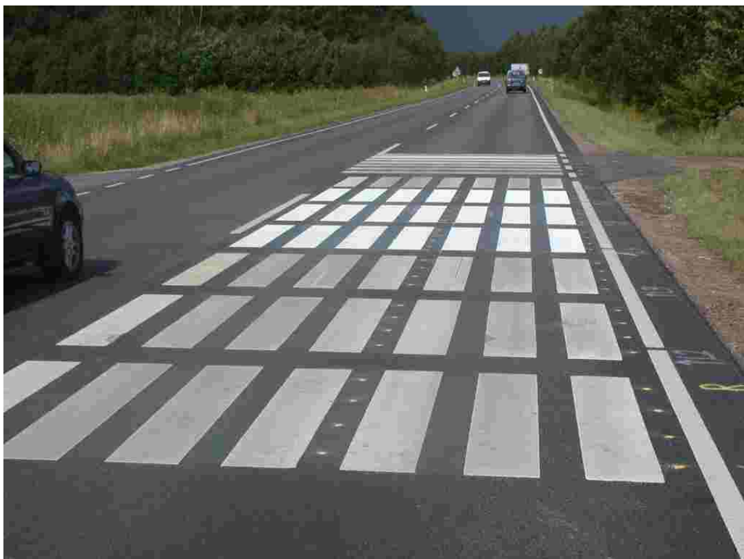
Figure 1.1: Example of a trial site with application in both the longitudinal and the transverse pattern (Denmark).
